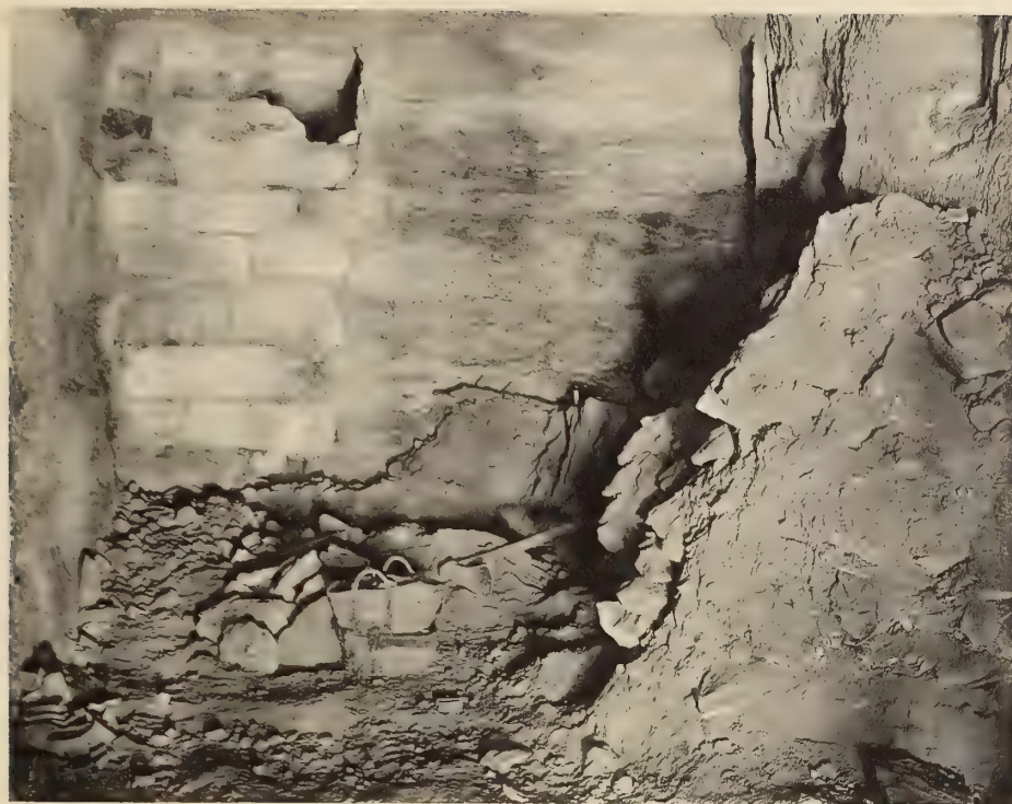
I. ENTRANCE CHAMBER UNDERGROUND.
